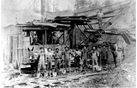
Workers pose at an excavation site with one of three Otistype steam shovels manufactured by John Souther and Company of Boston, Massachusetts, and in operation at Scotia. These excavators were brought in by Andrew Carnegie on the Lewisburg & Tyrone RR to speed production at the Scotia mines.
