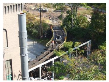
**Dismantling the Bellefield Steam Plant Trestle:** 2 years after the last coal hopper was shunted into the "Cloud Factory" by an aging Plymouth critter, crews on this brisk October morning are cutting up tracks and lifting crossties on the trestle. Within 2 days the trestle was gone, and Neville Street was soon widened to 2 lanes where the trestle had choked vehicle traffic to one lane for so many years. Photo by Patrick Altdorfer.
